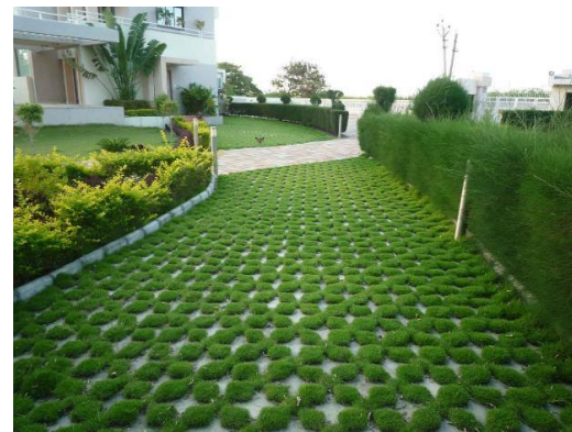
Infiltration pave way
