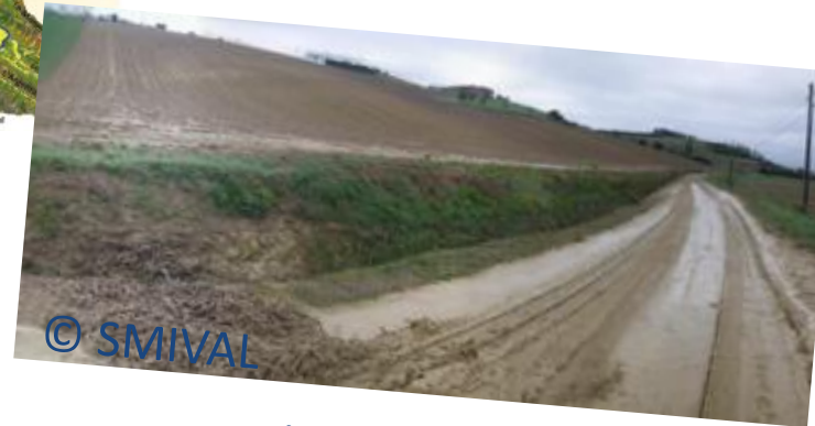
With erosion issues...
