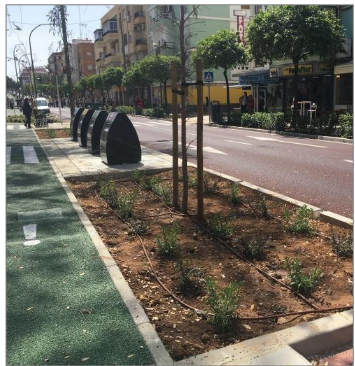
Permeable pavement and Bioretention system 2
