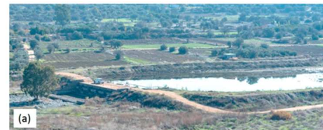
OROUNDA CHECK DAM (SOURCE: DJUMA ET AL., 2017)
