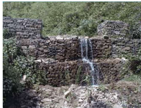
Gambion Check Dam (Source: Shrestha Et Al., 2012).
